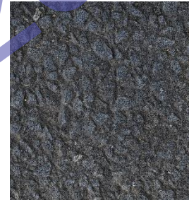
Dense Bitumen Macadam
